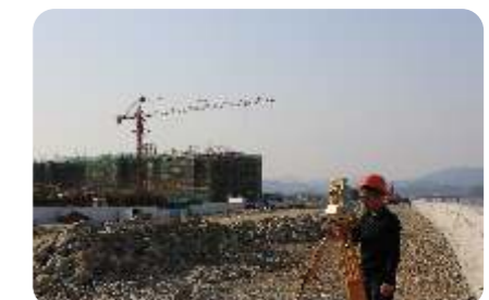
Road Program Calculates a complicated curve and a long distance route automatically, by defining the initial point, end point and curve parameters
